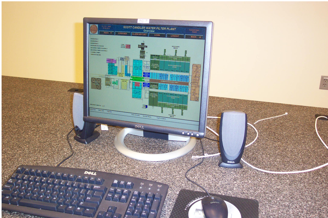
Figure 6-2 Example of a SCADA Workstation at a 25 MGD Water Treatment Facility
