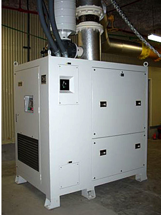
Figure 6-5 New Turbo Blower Installed at Lakota Wastewater Treatment Plant, WA
