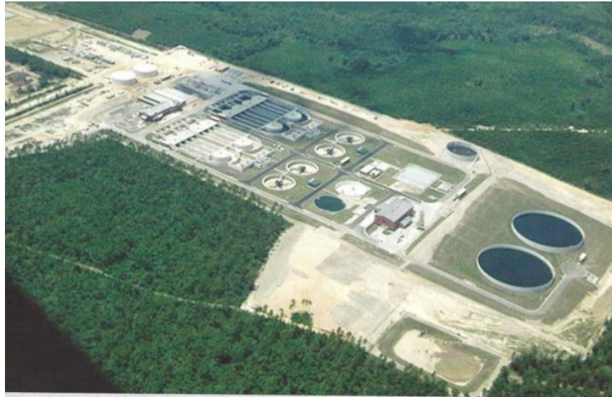
Figure 7-4 View of ECUA Central Water Reclamation Facility Site
